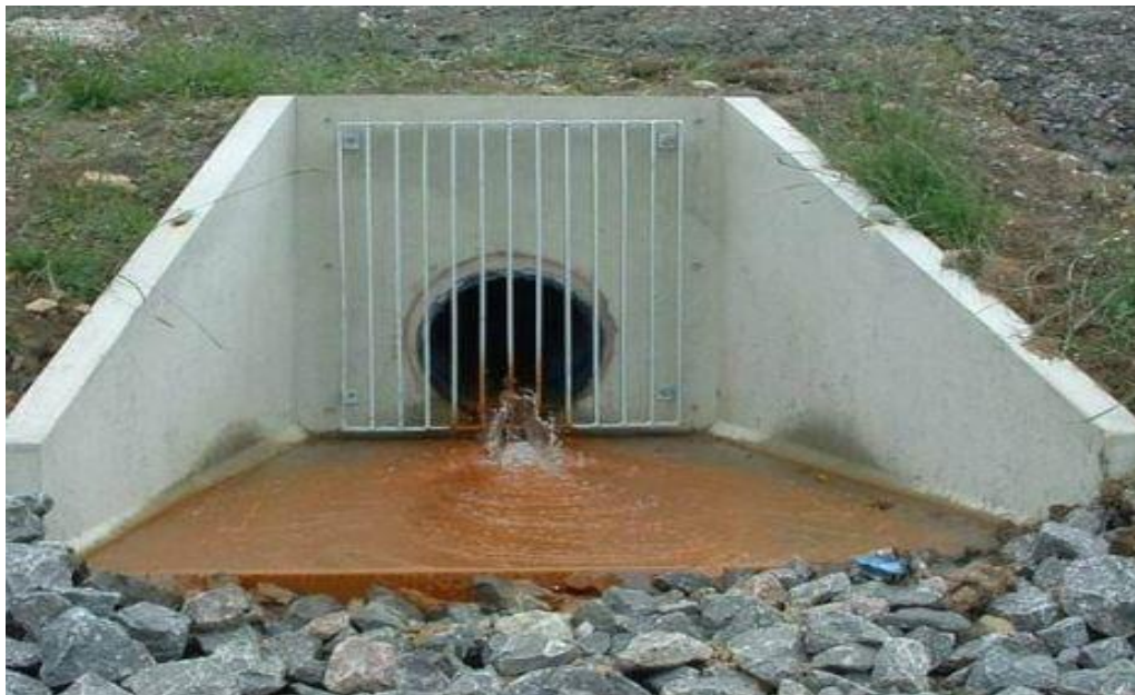
Fig 2:- Pipe Culvert with a filter
