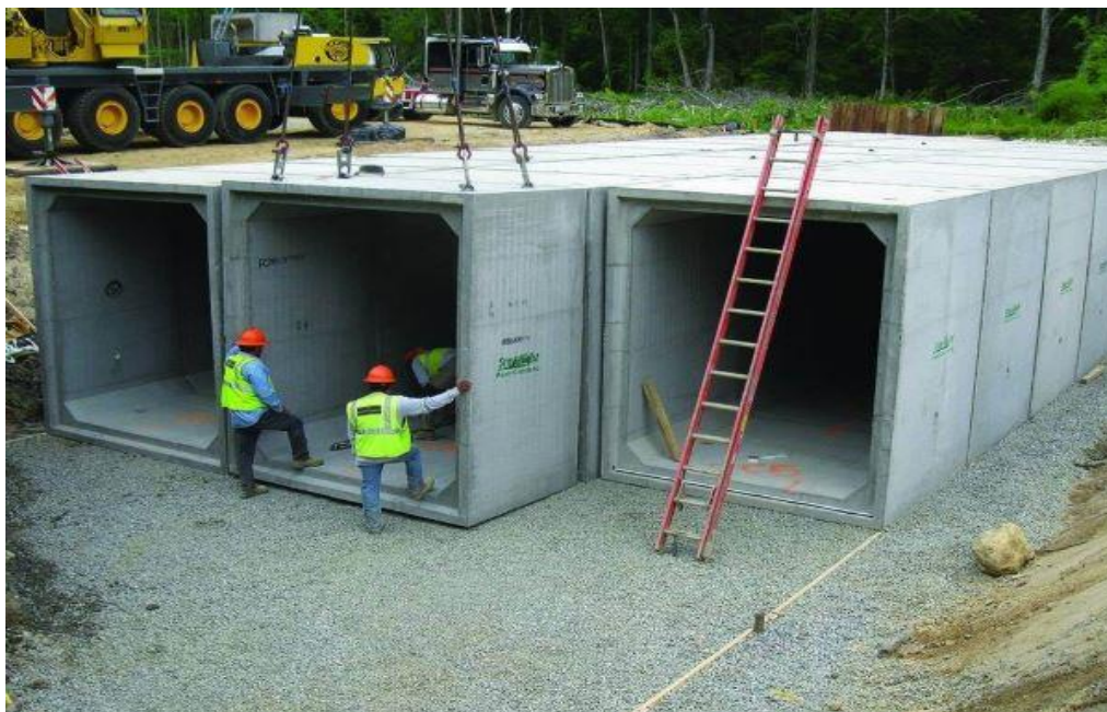
Fig 4:- Box Culvert
