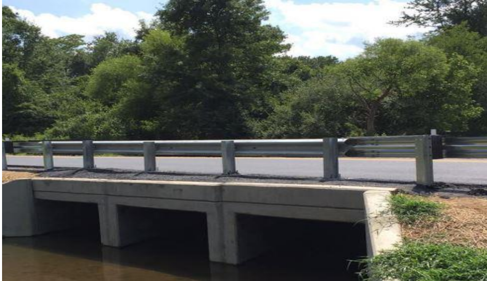
Fig 7: Rcc Solid Slap Culvert
