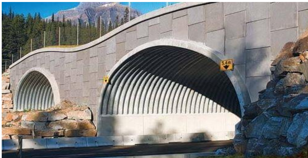
Fig 10: Steel Arch Culvert
