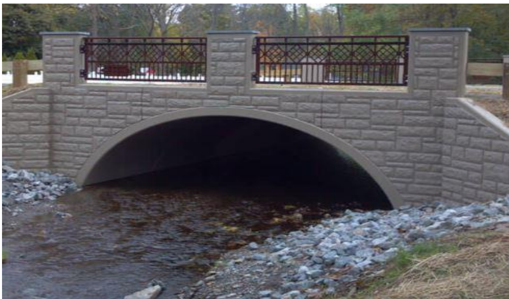
Fig 6:- Pipe arch Culvert with a small channel
