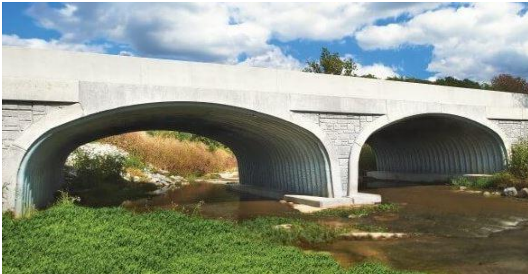
Fig 9: RCC Arch Culvert
